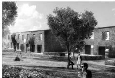
Residential refurbishment Ryhaven Aarhus
