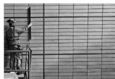
Interior works Cph Metro Copenhagen
