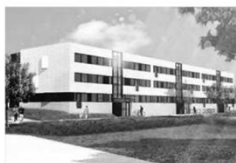
Residential Refurbishment Åbyhøjgård Aarhus
