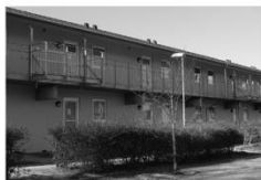
Residential Refurbishment Byengen/ Nordengen Kokkedal
