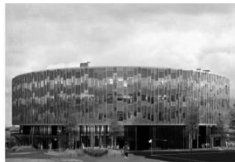
Construction of school Kalvebod Fælled Skole Copenhagen
