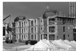
Residential Construction Tuujuk Nuuk
