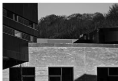
Construction of psychiatric ward on PPP basis Vejle Sygehus Vejle
