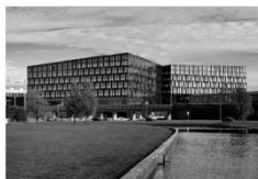
Construction of head office Nordea Ørestaden
