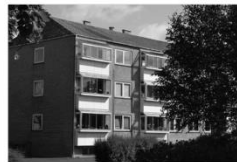
Residential Refurbishment Stadionkvarteret Glostrup
